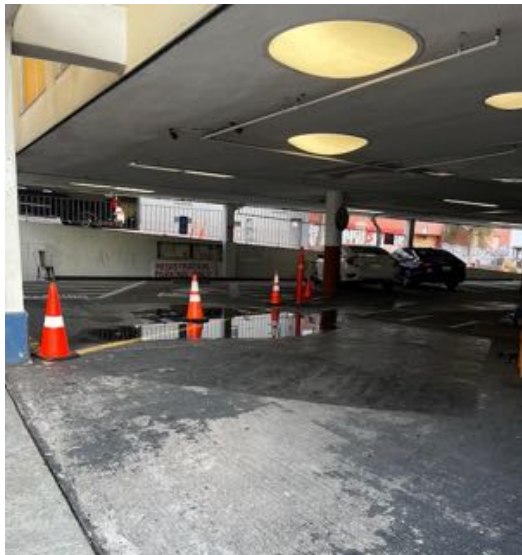
Building piping as seen at hallway ceiling - copper water supply, cast iron waste
