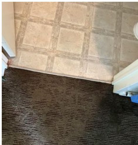
Carpet flooring and bathroom sheet vinyl flooring
