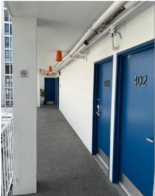
Hallway surface and railing
