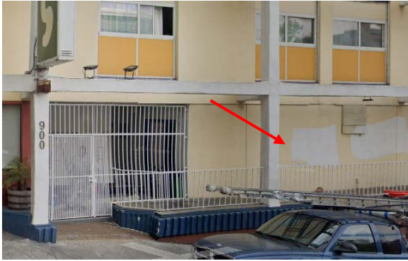
Figure 1: Photo of exterior taken May 2022 (Exhibit 11).
