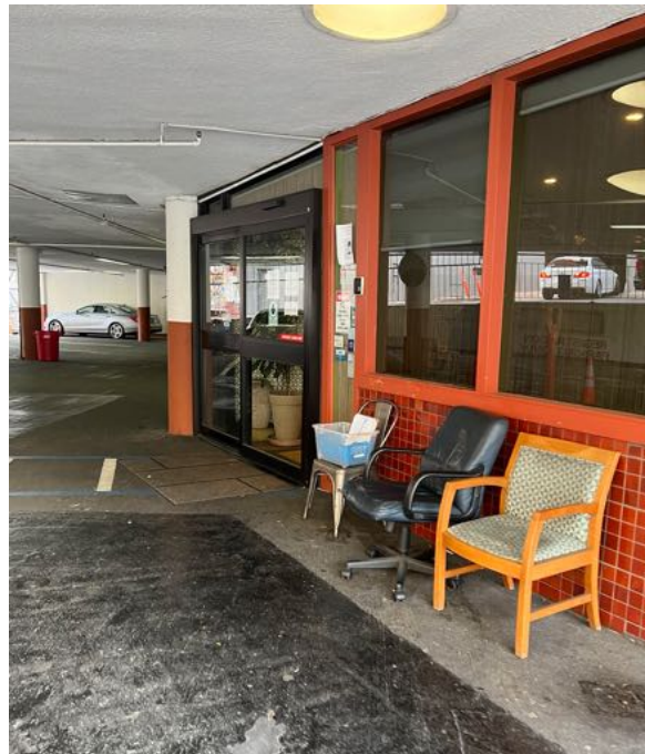
Main entry door at garage entrance on Franklin Street
