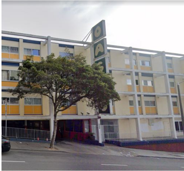
Driveway entrance and project sign
