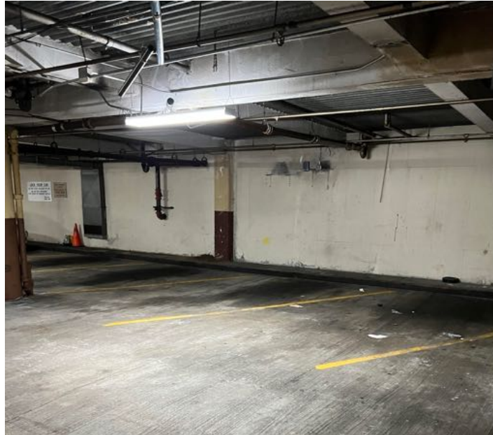
Upper and lower garage
