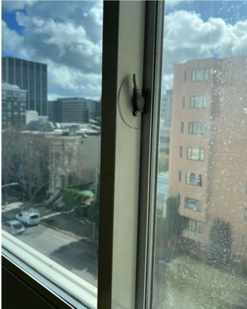
Sliding window at Unit 408
